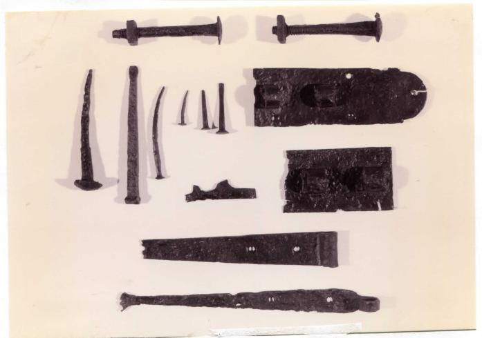
Architectural hardware: hinges, sliding bolt locks, handwrought nails and spikes, bolts
